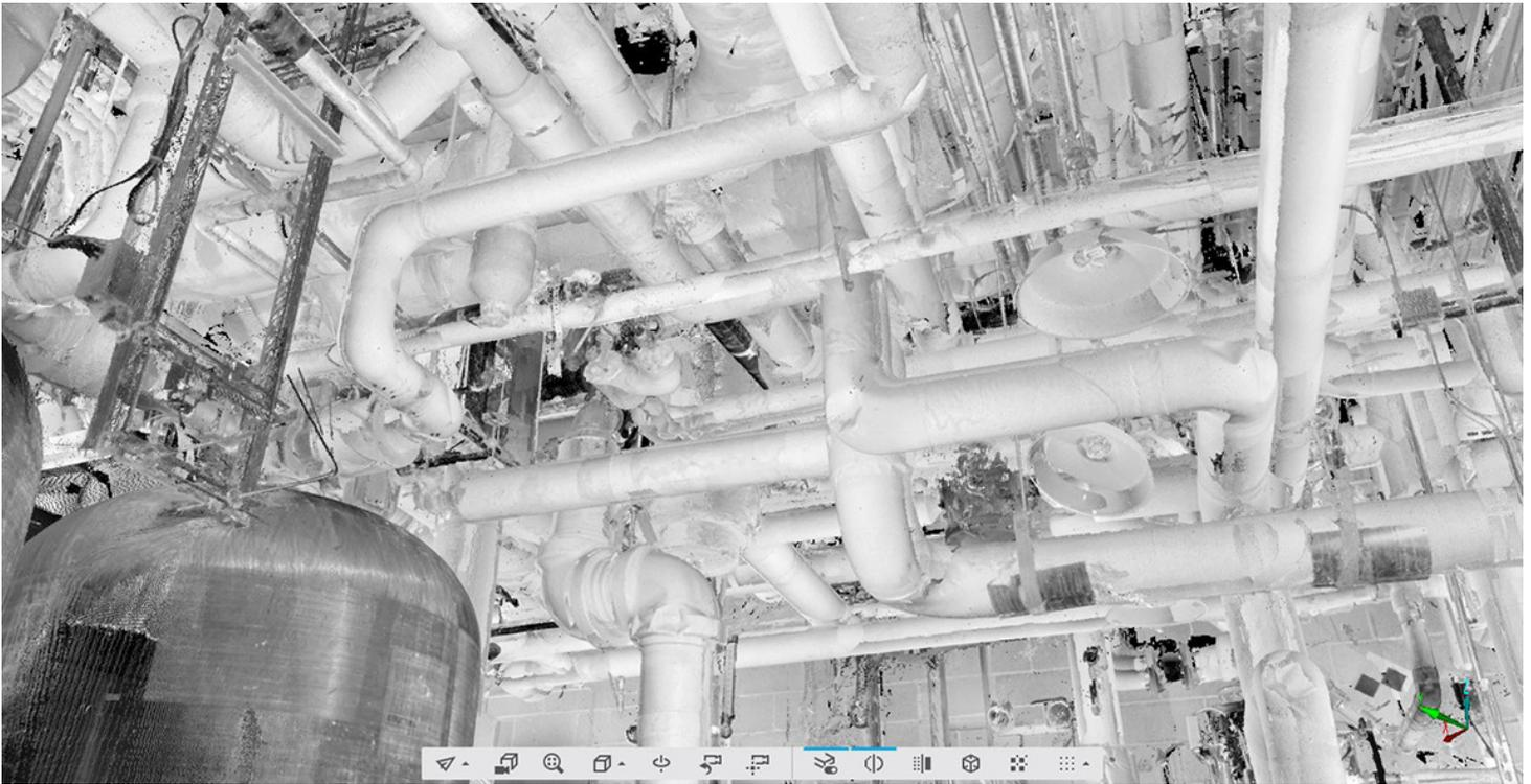
To accurately capture the extreme congestion of the mechanical room, J Brown pushed the FARO Laser Scanner up through layers of pipe.
